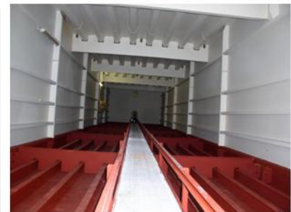
Other areas under the bridge that also needs maintenance are what are known as "boxes". They are actually large metal rooms and one would get the impression that they are standing in the hull of a ship or submarine. The red coating pictured is actually a "lead based" paint. The Pneumatic MBX Bristle Blaster with the dust extraction unit was the ideal solution in this case
