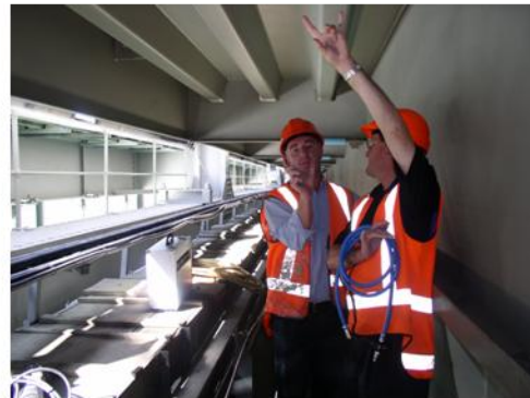
Keith (left) from TBS and William from Syntech in discussion of what is required. Keith explaining the width required
